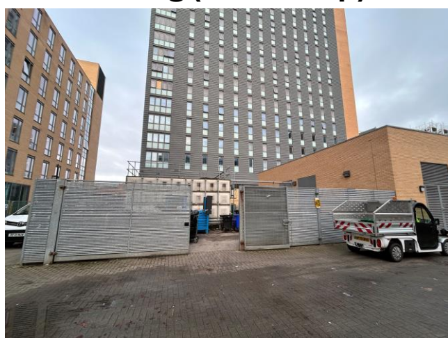
Waste yard for Alan Turing building (46 on map)
